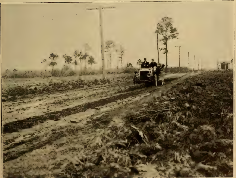
Near Harrington, Delaware—where real ruts are to be found.
